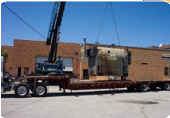
Removing the old, inefficient boiler
